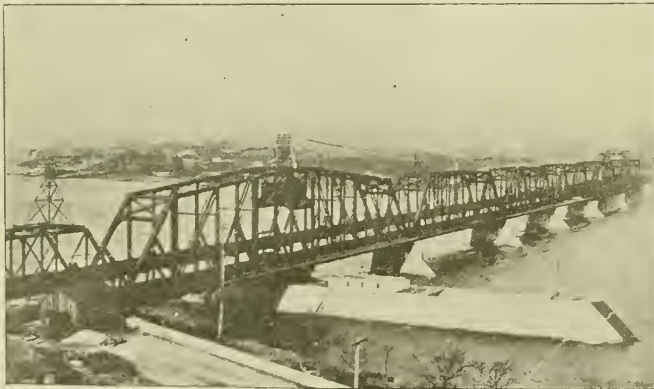
The New Rock Island Bridge.
